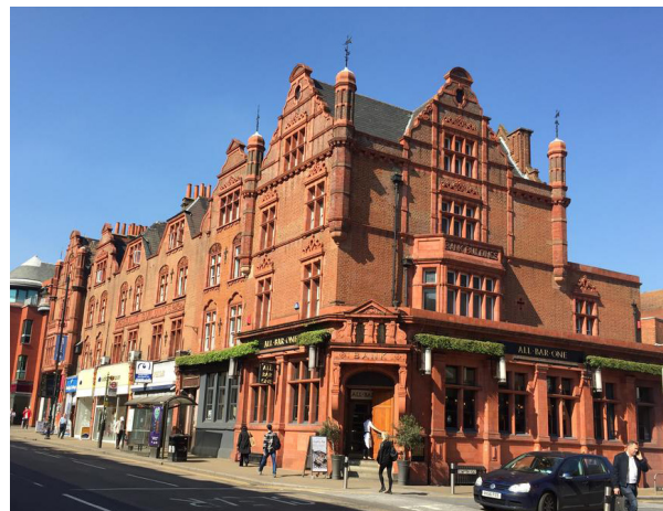
28 Bank Buildings, Wimbledon Hill Road
